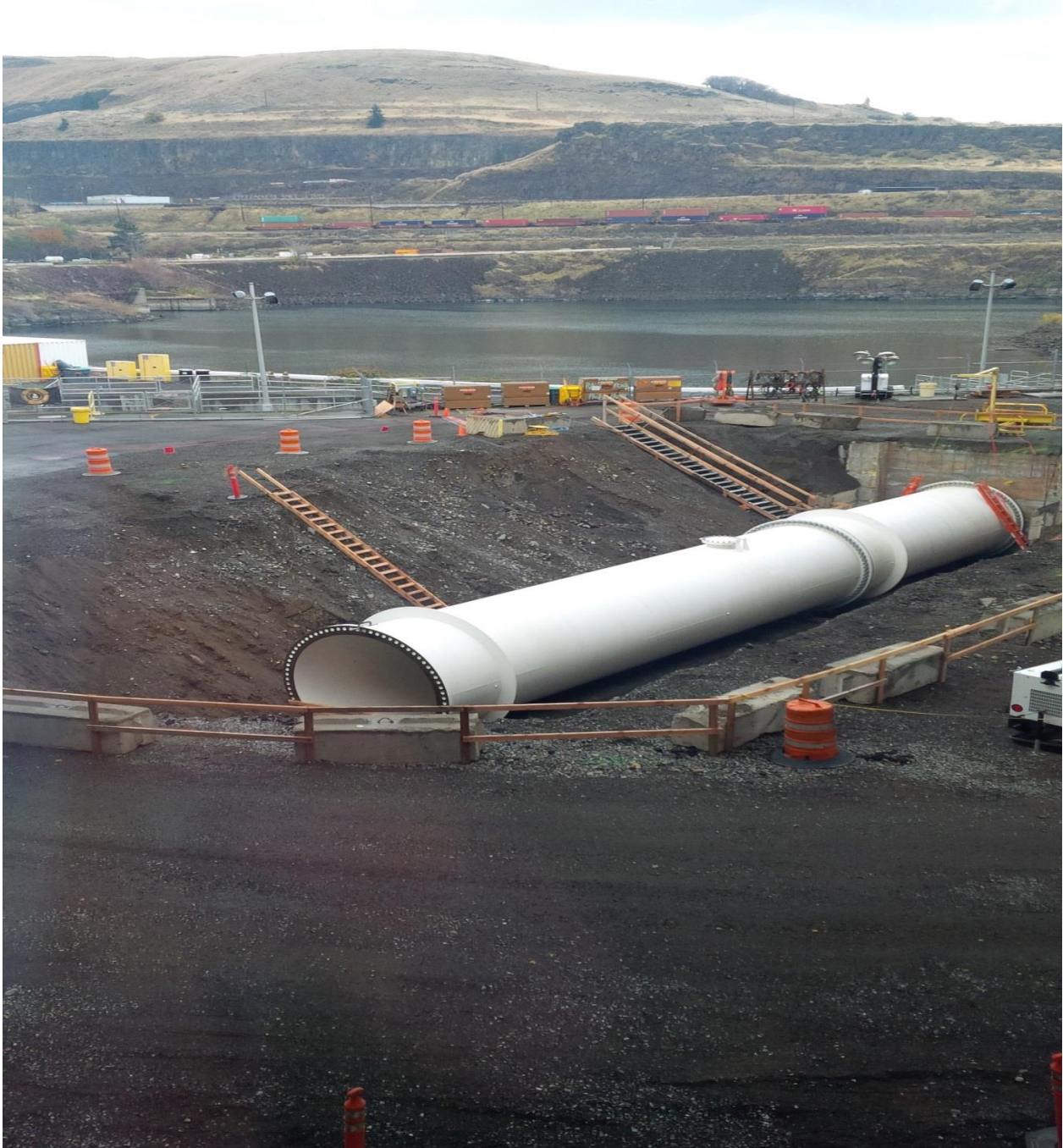
Getting closer...shiny new section of AWS pipe installed.
